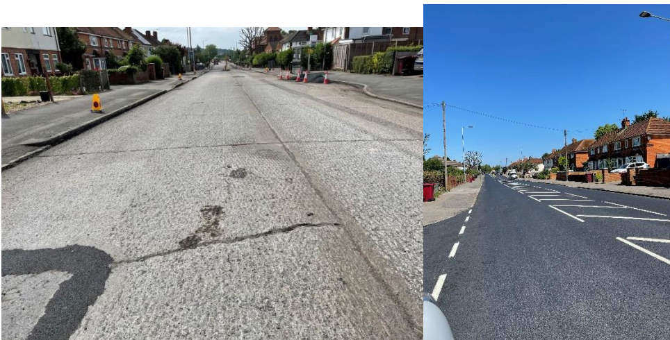
Northumberland Ave Before & After
